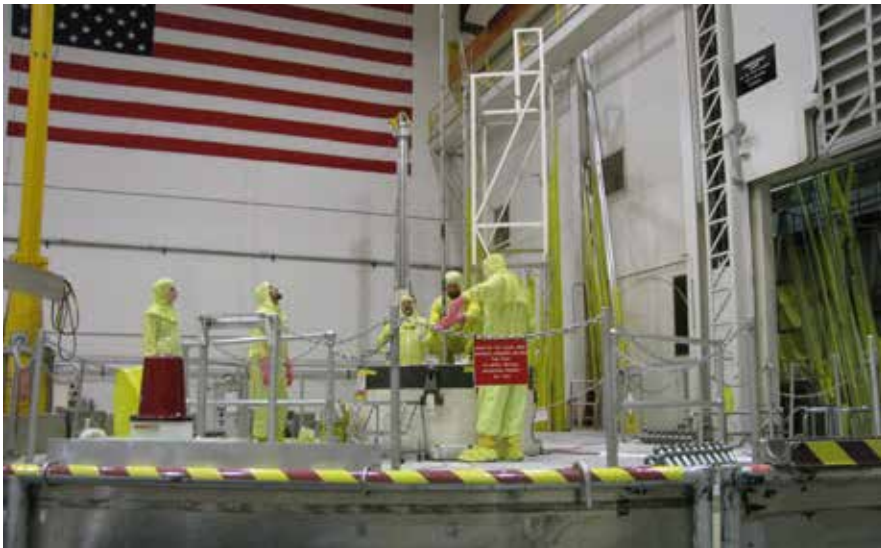
Figure 2. Installation of ATF-2 in the Advanced Test Reactor Loop 2A in the Center Flux Trap.
