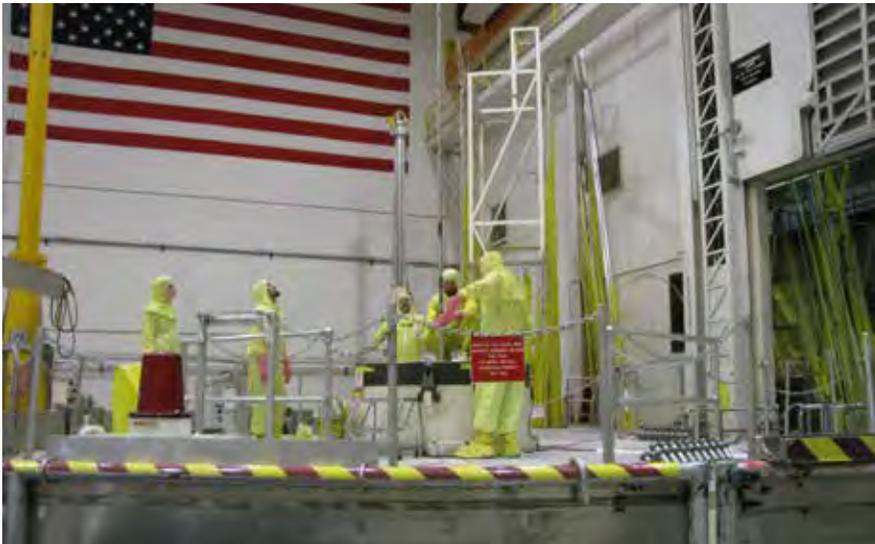
Figure 2. Installation of ATF-2 in the Advanced Test Reactor Loop 2A in the Center Flux Trap.
