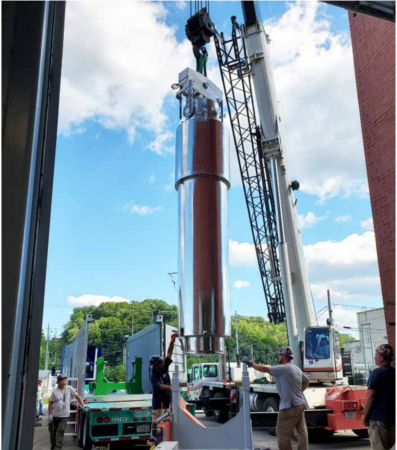
Figure 3. The cask containing Westinghouse ATF and high burnup LTRs is unloaded at ORNL
