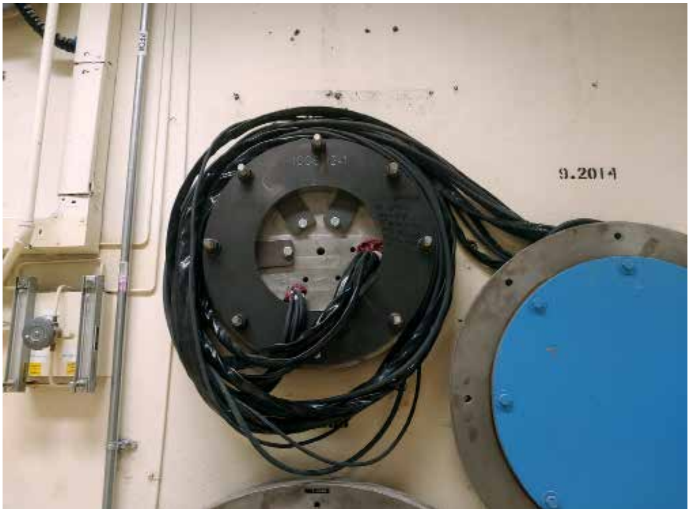
Figure 1. New HFEF feedthrough installed to support refabrication/welding equipment
